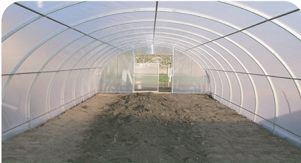
Walk In Tunnel House
